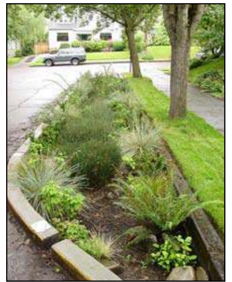
Bioswales such as this one collect stormwater from our streets, preventing neighborhood and basement flooding, reducing pollution in our rivers, calming traffic, and saving ratepayers money. © Mike Houck
